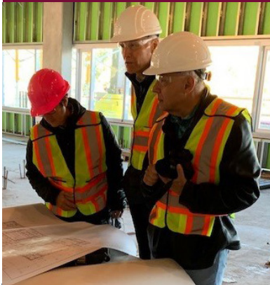
Judges visit Abbotsford Law Courts during construction
