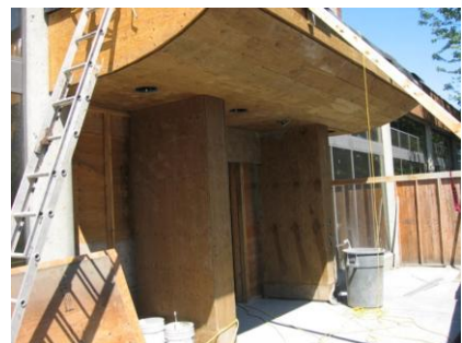
The entrance begins to take shape
